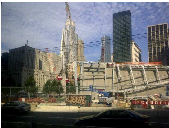
Selects have arrived at Battery Park...
